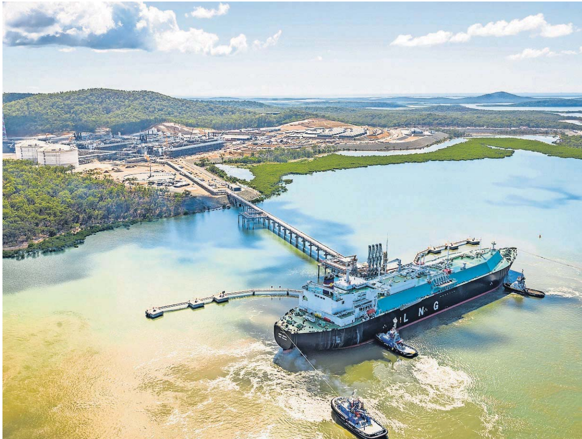
Maintenance contractor UGL has agreed to give workers at the Santos-led GLNG project on Curtis Island in Queensland a 7.5 per cent pay rise. Below: Steve Knott says employers are being squeezed on multiple fronts.
